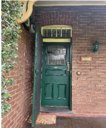
Figure 4.7 The original timber and glass panelled door with leadlight.
